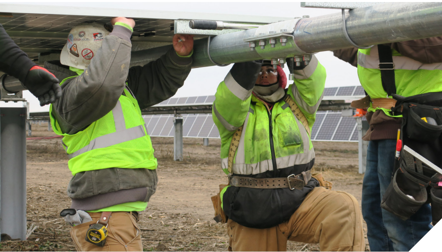
Workers on a solar installation project - Mid-America Carpenters Regional Council
